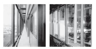
A double-skin energy-saving curtain wall is an outer building structure consisting of an outer curtain wall and an inner curtain wall. It is also known as a dynamic ventilation curtain wall, hot-channel curtain wall and respiration curtain wall. Compared with conventional curtain walls, double-skin curtain walls can effectively improve the thermal insulation of the outer building structure, indoor ventilation, sound insulation and daylighting.
