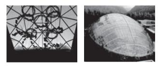
A skylight, which consists of transparent panels and its supporting system, is a roof system that has a horizontal angle of less than 75 degrees. It provides natural lighting for the building and serves other related functions. The transparent panels are usually made of glass, polycarbonate sheet and transparent membrane materials.
