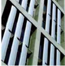
A shading system is used to shield a building from excess sunlight. It helps to improve the energy efficiency of a building by reducing the amount of air conditioning required in the building. We have applied intelligent control technology to some of our shading systems, which can automatically adjust its position in response to the sun's path.
