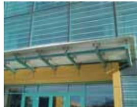
A canopy system is the outer structural component of a building which is located at the entrance and exit of the building, serving the function of shielding the building from wind, rain and sunshine. Under the canopy is a semi-open space which is the exchange and transition buffer zone between the inner space and outer space of the building. The canopy system is an important part of a building's outer decoration system, which highlights the whole building.
